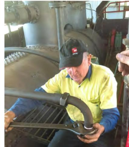
A second trip was cancelled when a possible fault was observed in the boiler feed water piping. Work is currently proceeding on the replacement.
